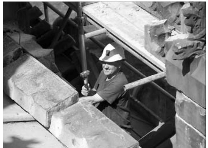
Some of the blocks at the top of the wall had to be completely replaced - you can spot the new blocks from below. Each took more than 3 hours to carve!
